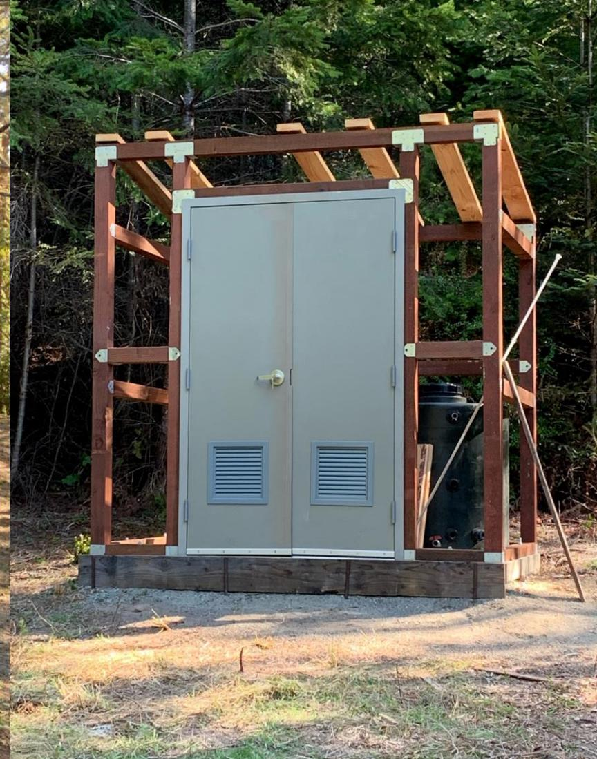
Fireproof doors were installed, and the crew completed the enclosure for the mini-treatment plant at Tank 2. The crew also installed a back-up generator.
