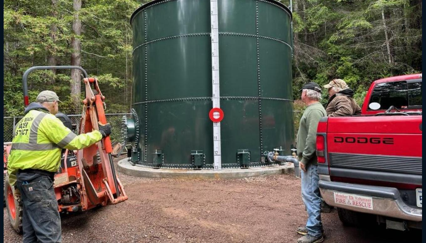
Construction of Tank 5, plumbing and electrical connections between Tank 5, Well 5, and Tank 4 were completed in early December. Grading the site after trenching for plumbing and electrical connections was completed the second week of December, and Tank 5 was filled with water and brought online soon thereafter.
