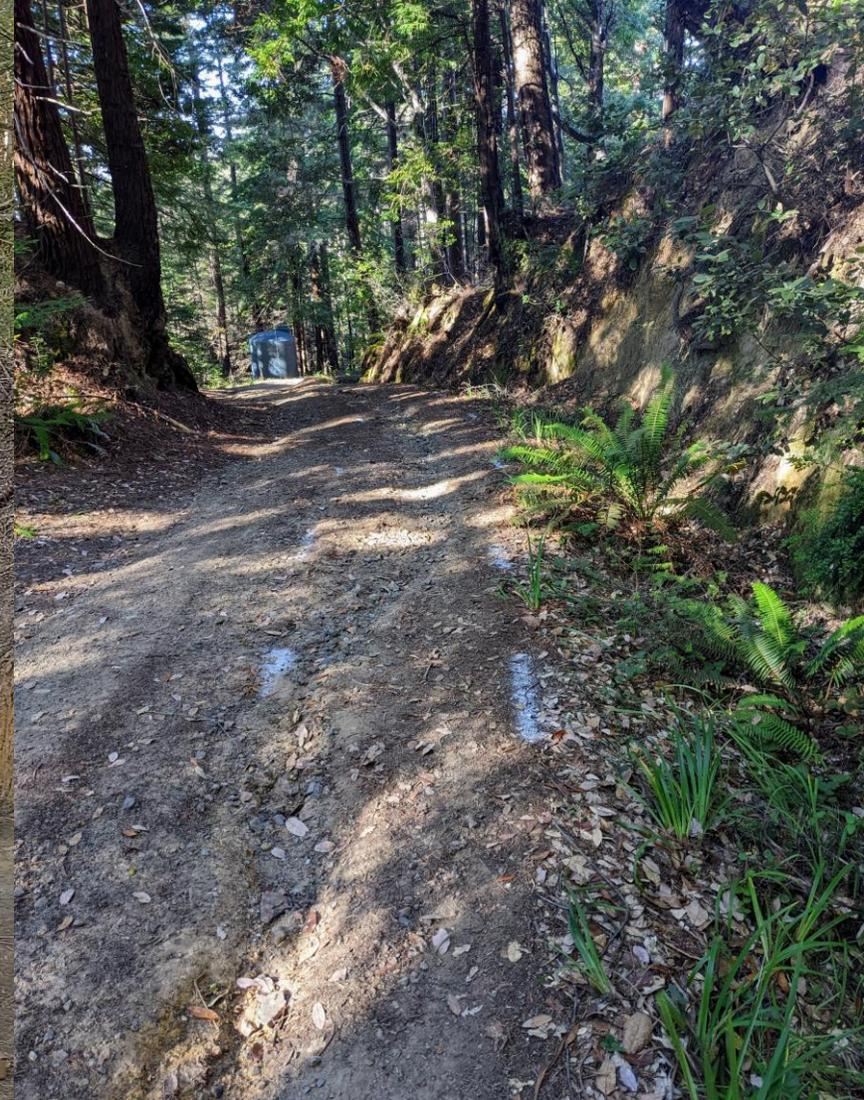
The Tank 2 site was cleared and prepped for delivery of the new cover and the roadway was marked for trenching.
