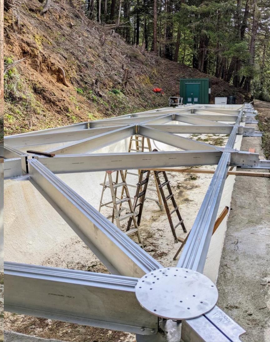
The Operations crew installed the girders for the new Tank 2 cover.
