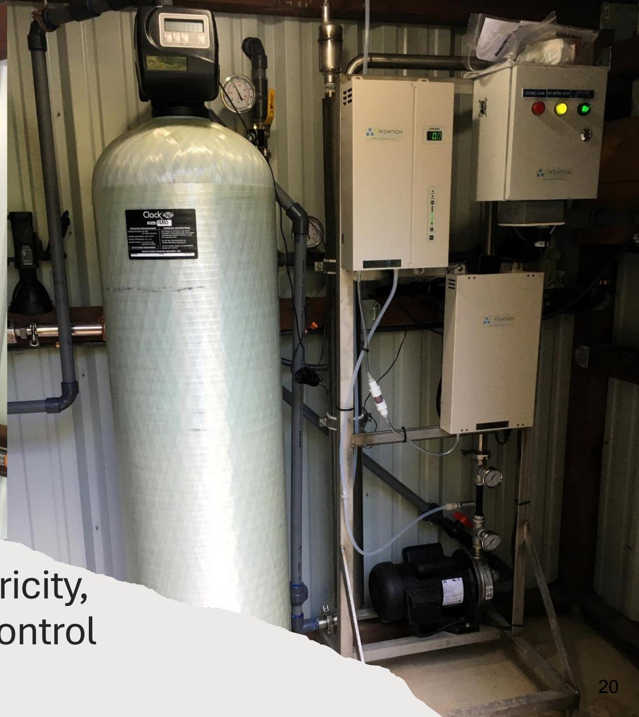
Once Well 2 & Tank 2 sites had electricity, the ozonator, filtration system, and control panels were installed.
