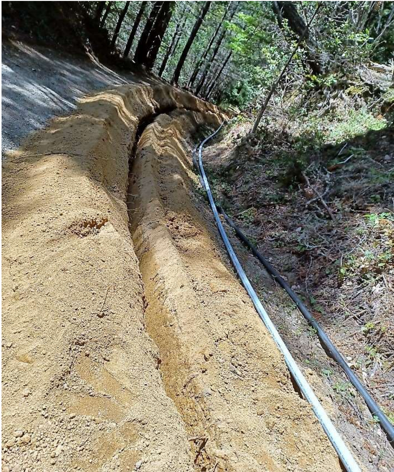
Task 3-2 – Well 2 Activation: Trenching for water line and electrical from Well 2 to Tank 2:
