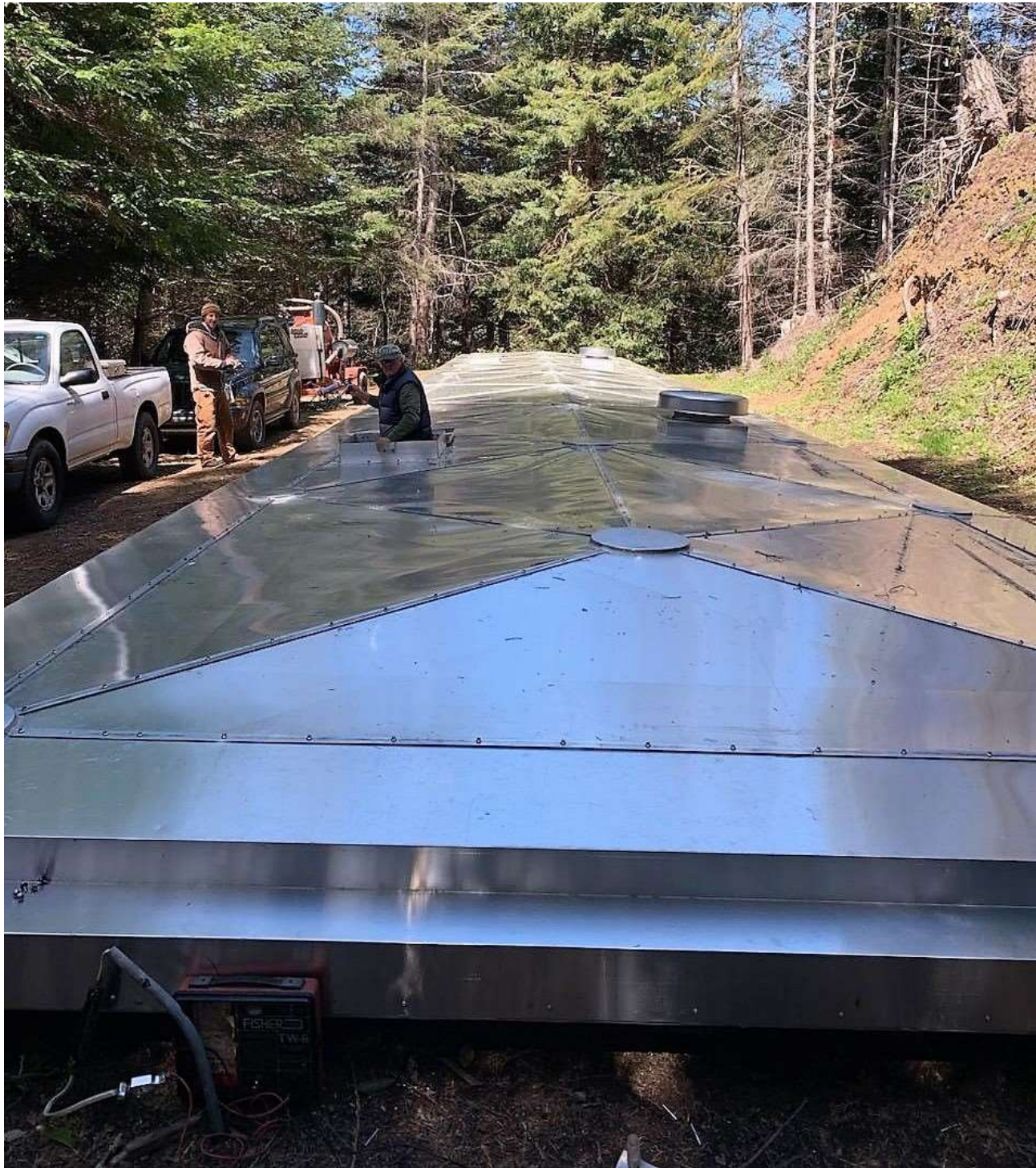
Task 3.3 – Tank 2 Restoration: Metal roof – vents installed, and tank sealed:
