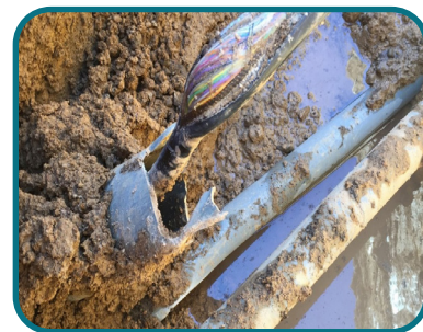
High-risk thin wall PVC pipelines with glue joints, prone to failure, located next to electrical lines.
