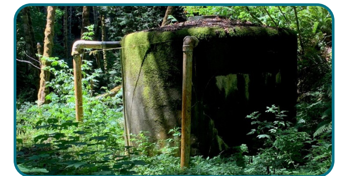
Circa 1983, 10,000-gallon concrete tank. Replace with epoxy-coated steel tank. Existing tank is cracked and weak, posing contamination risk.
