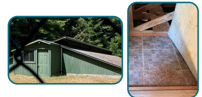
Circa 1989 - Tank 4: 125,000-gallon concrete tank. Wooden truss structure covering tank is deteriorating, infested with termites and carpenter ants, and vulnerable to contaminants.
