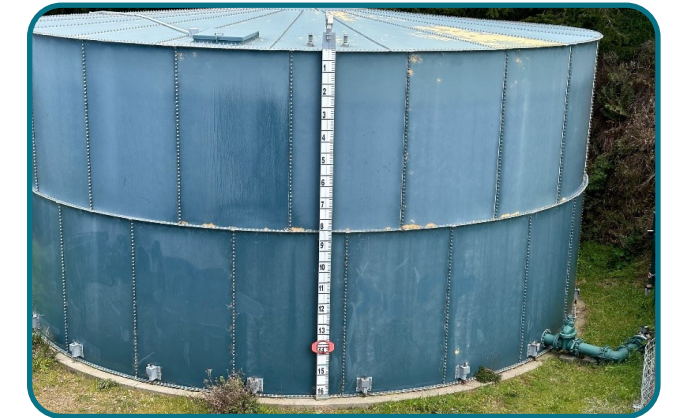
Tank 3: Recoat the 84,000-gallon steel tank with 2-part epoxy paint to address exterior coating damage and prevent reduced lifespan.
